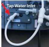
2. Install shortest part of tubing at the Tap Water Inlet - make sure the arrow on the Sediment Filter points towards the TAP WATER INLET.
